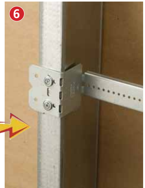
6. Install TSGB to stud with SMS8 low-profile screw.
