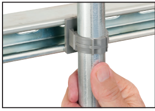
5 Secure installation of conduit to strut.
