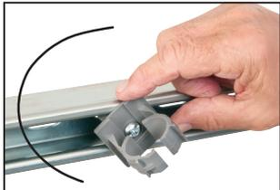
2 Twist QuickLATCH to seat clip in strut.
