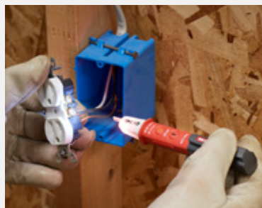
Test wires for AC voltage
