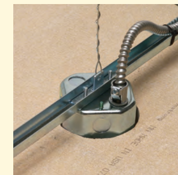
4 Cable pulled through cable connector (not supplied).
