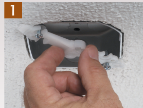
1 Back the screws out enough to slip the bracket on.
