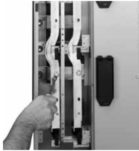
Field Phase Balancing
