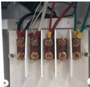
Copper Busbar with Ratings from 250 to 500 A
