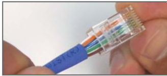
Insert wire pairs into plug
