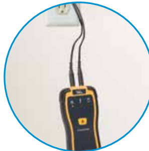
Traces on de-energized circuits
